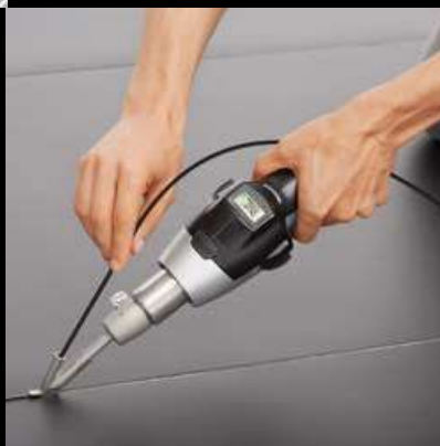
▼ Welding linoleum floor HG 2620 E
