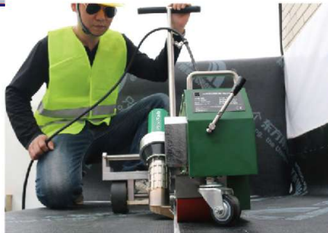
Welding Modified SBS by Flameless Method PFE-WP2
