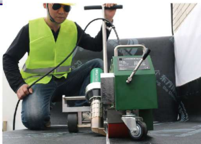
Welding Modified SBS by Flameless Method PFE-WP2
