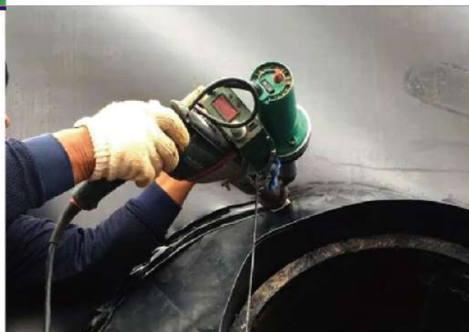
HDPE Membrane Welding PFE610A
